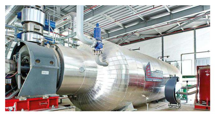
Turboden has signed an agreement with Centrale del Latte di Brescia for the installation of the world's first high-temperature cogeneration ORC plant – Steam & Power Organic Rankine Cycle System (photo Turboden).
