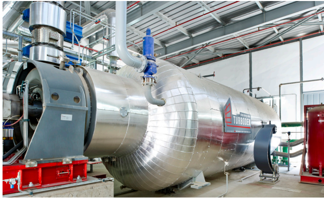
2 MWe Turboden ORC system at an Italcementi cement plant.
