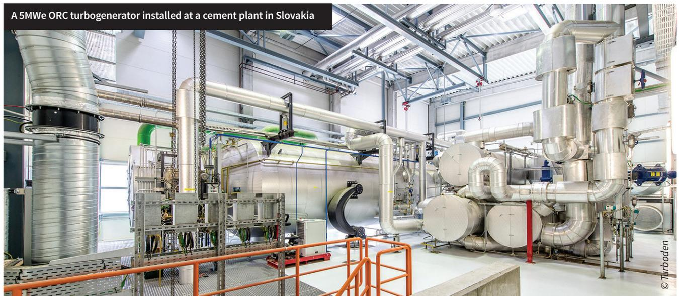
Over the past decade, organic Rankine cycle (ORC) technology has emerged as a viable and safe alternative to the classic steam Rankine cycle as a waste heat recovery (WHR) technology for the cement industry. Technological improvements, increased competitiveness, and the general tendency towards a greener and more sustainable environment supported by governments across the world have made
